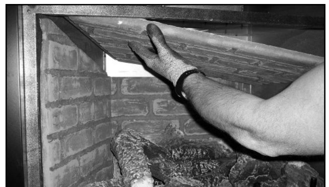
Figure 7.21 Remove Top Refractory
